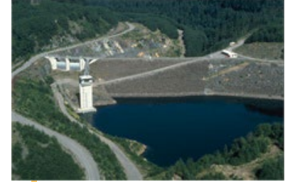
Howard Hanson Dam
