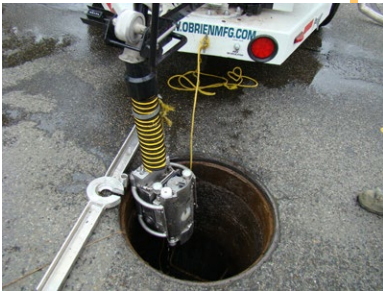
Environmental Services inspects its stormwater pipes using a hydraulic-powered video camera
